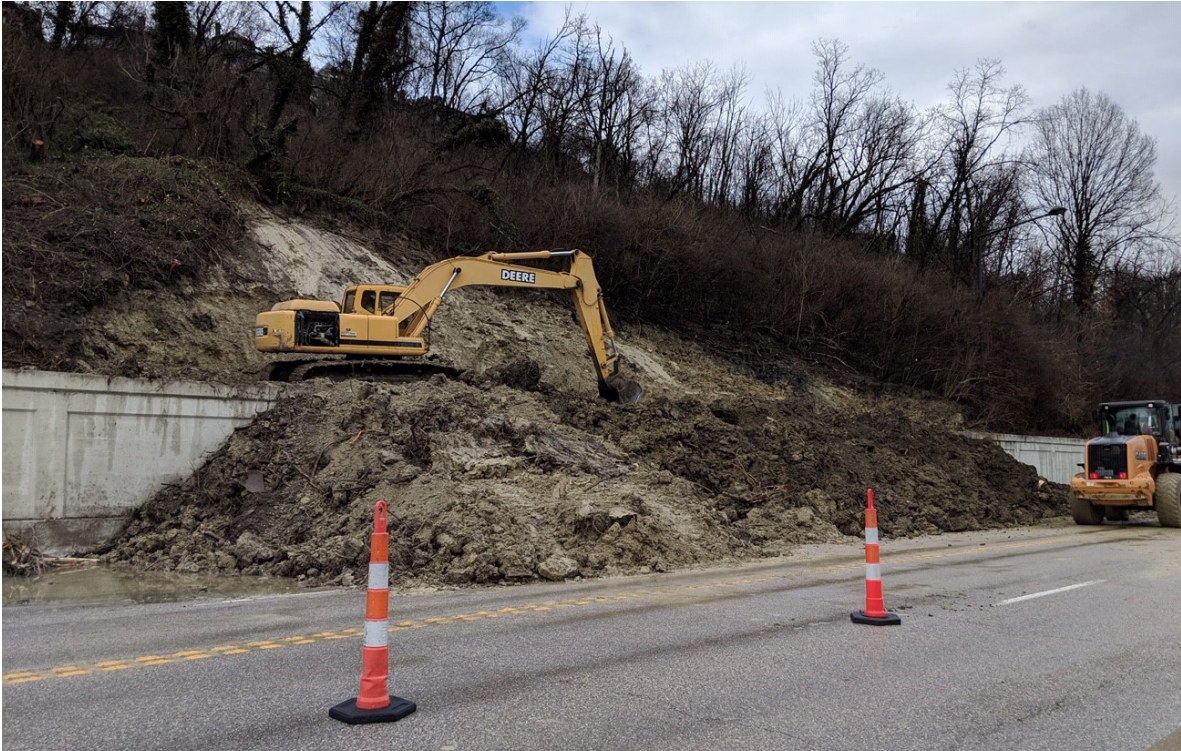
Figure 24: Landslide removal Area 9, March 21, 2019
