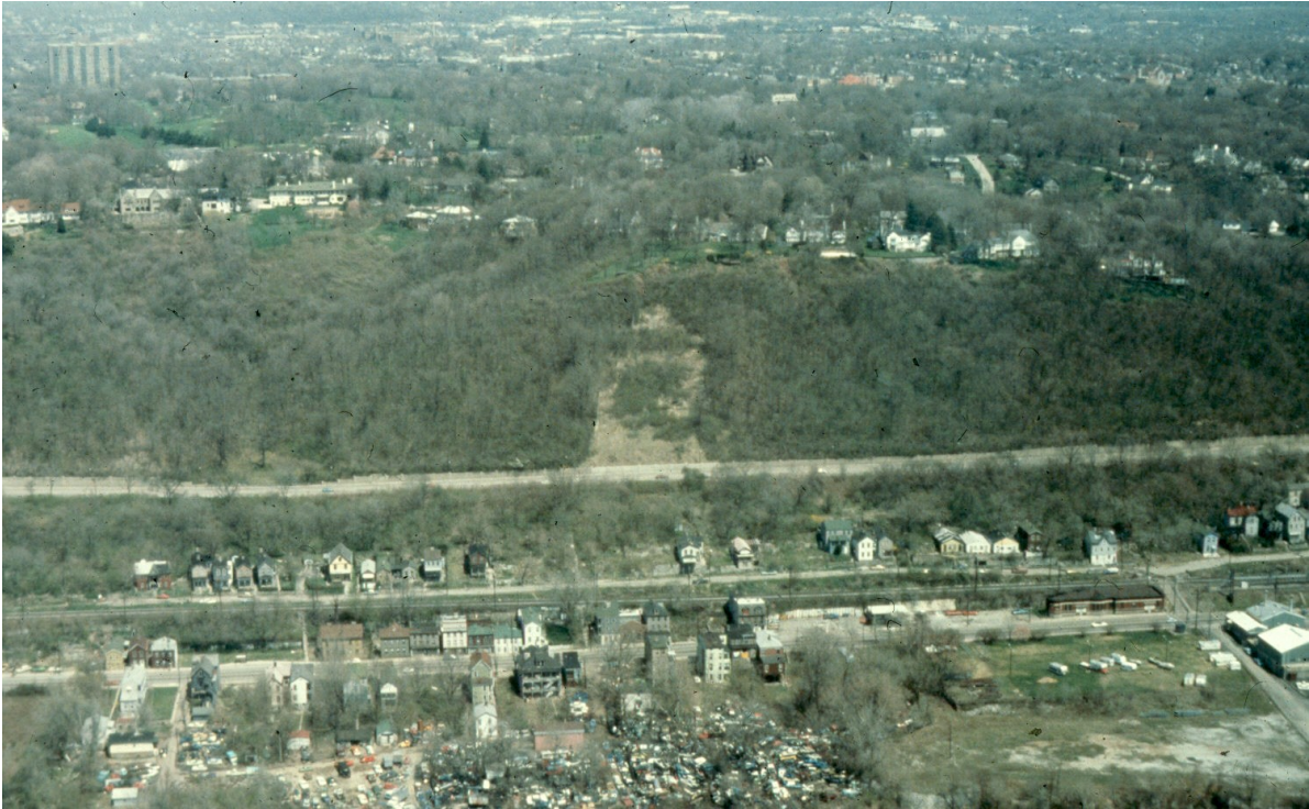
Figure 3: 1975 landslide west of Audubon
