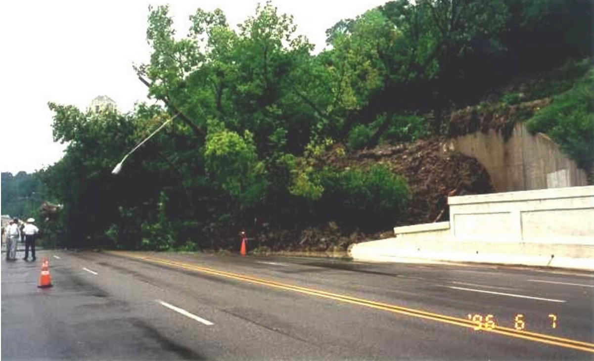
Figure 5: 1996 landslide at 2110 Columbia Parkway
