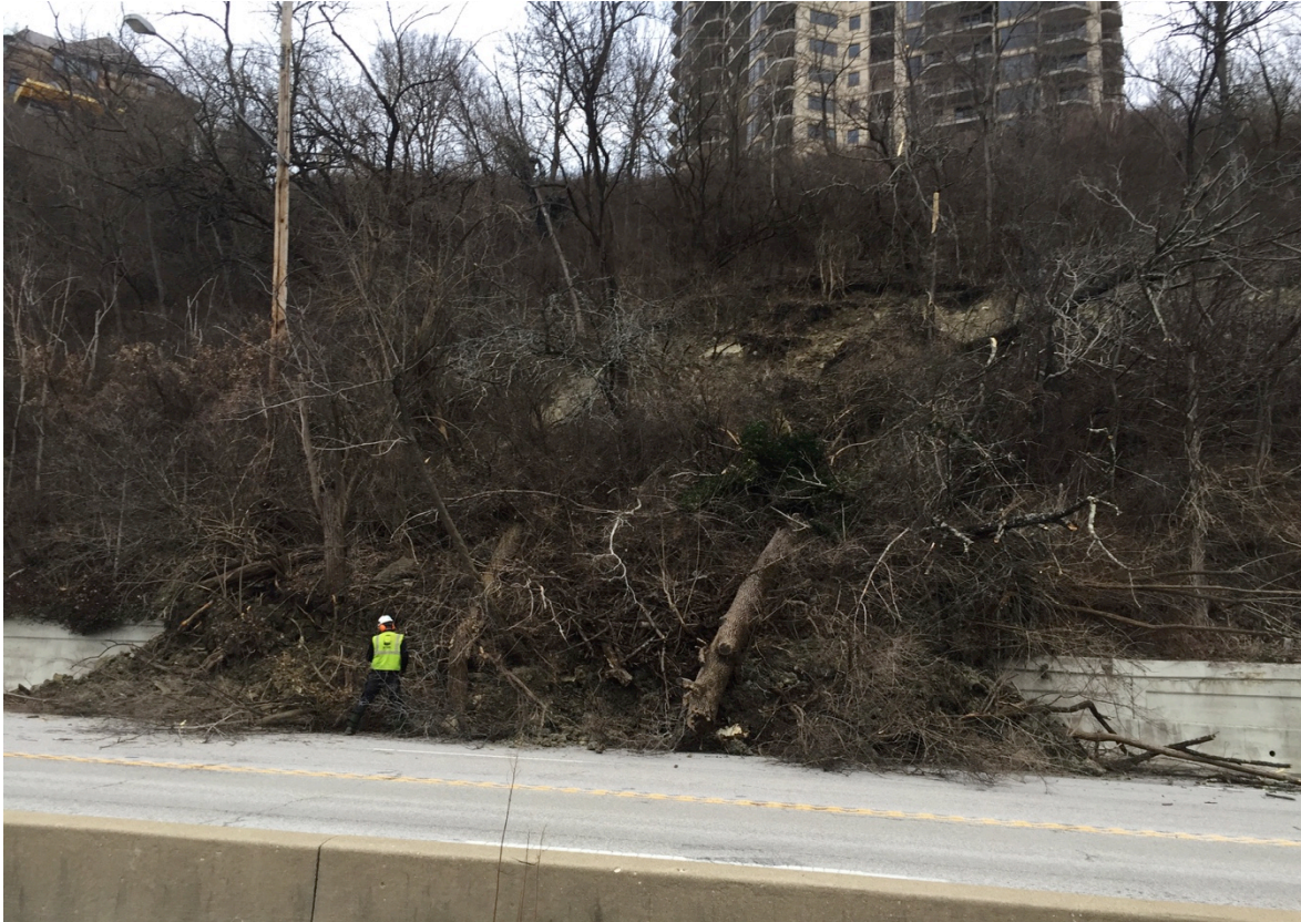
Figure 7: Jan. 29 th 2019 landslide on Columbia Parkway 1,000 ft. east of Kemper Lane
